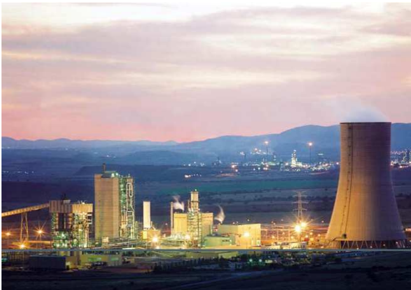
Figure 1. Elcogas IGCC power plant.
